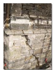
Stonemason **Richard Strachey** carried out the majority of the stonework. The urgent work on the porch involved dismantling and rebuilding the random-rubble merlons (for the less technical, that's the 'sticky up bits') and a lot of the wall below them. The merlons had been dangerously loosened by movement and weather over 400 years. In the
