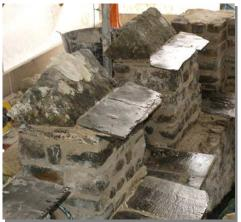
end the damage was worse than feared and the walls had to be taken down to the string course below the roof line. The SW corner *(above left)* had settled significantly since it was last repaired in the 1870s, perhaps because of the vault placed below the porch in 1804.
