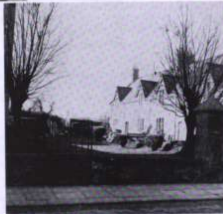
13 Lower Almshouses—Pilton Street
