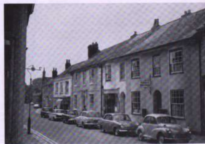
2 Pilton Street, Reform Street Junction
